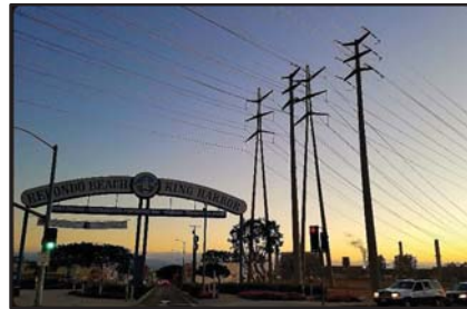
Remove utility visual blight
