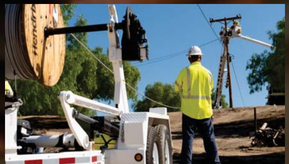
Above photos: SCE crew installing insulated wire
