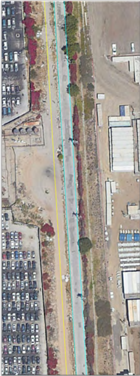
Blinn Avenue Widening
