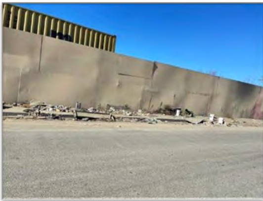
South Side of Q Street
