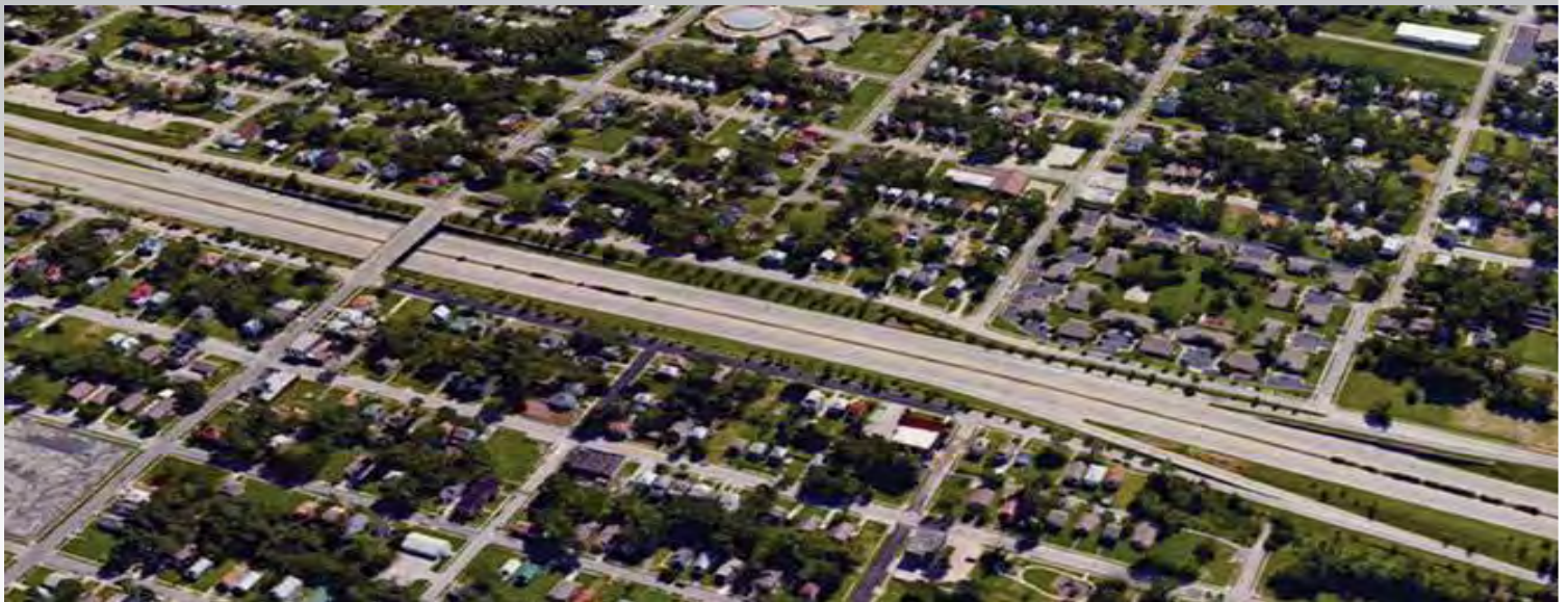
Completed in 2002 through Ivanhoe neighborhood (photo courtesy of @JSchnauzer via twitter)
