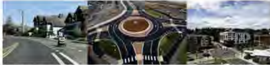
Visual examples of Complete Streets - All depict roads that have separated bicyclist and pedestrian facilities. The first image is a linear segment (in Port Townsend), the second (in Walla Walla) and third (in Bothell) are aerial views of a round about and signalized intersection.
