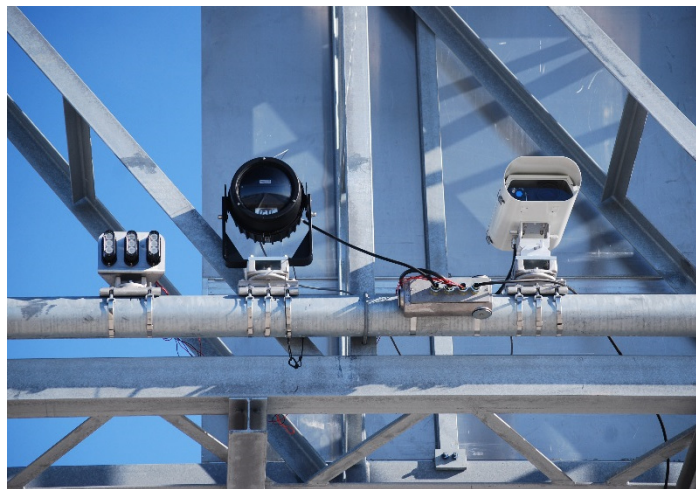
Figure 8-4: Example License Plate Recognition Camera and Illumination Equipment
