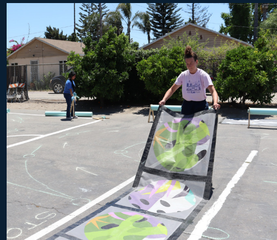
The project team built a temporary creative crosswalk and a separated bike lane.
