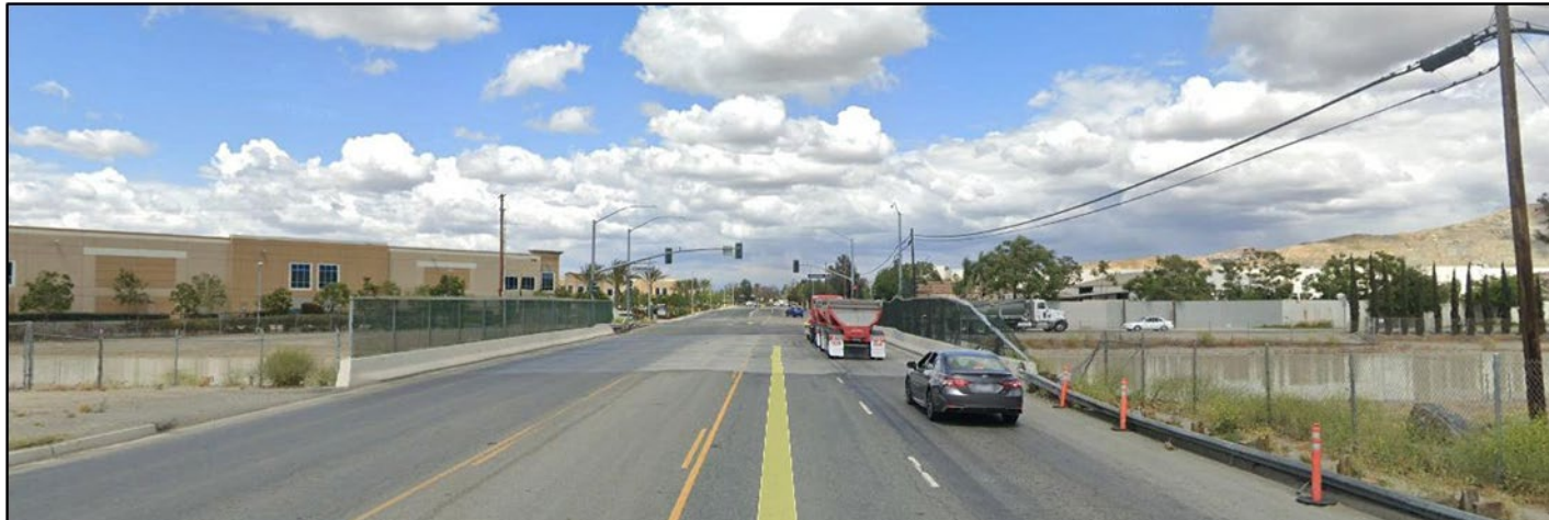
Figure 4: Photos of Existing Conditions at Bridge (looking east)
